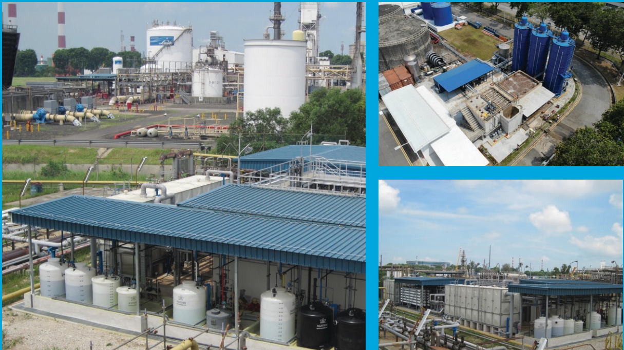
Figure 3: From left to right: (i) overview of the effluent treatment recycling plant, (ii) view of the fibre-reinforced polymer tank and the MF filtrate/RO feed tank, and (iii) close-up of the pressure vessels containing the RO membranes.
