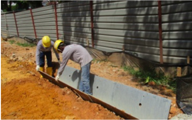
Use 2 manpower to install - overlapping.
