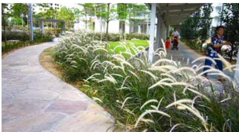
Fig. 10.13.2 The Peak @ Toa Payoh (Left). Fig. 10.13.3 Bioretention swales near Central Plaza (Top right). Fig. 10.13.4 Bioretention swales along walkways (Bottom right).
