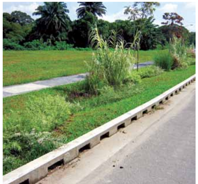
Fig. 4.16 Bioretention swales along Margaret Drive.
