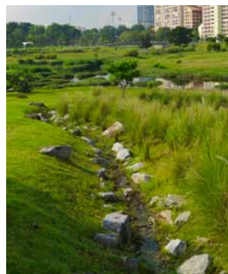
Fig. 10.5.4 Vegetated swales in the park.
