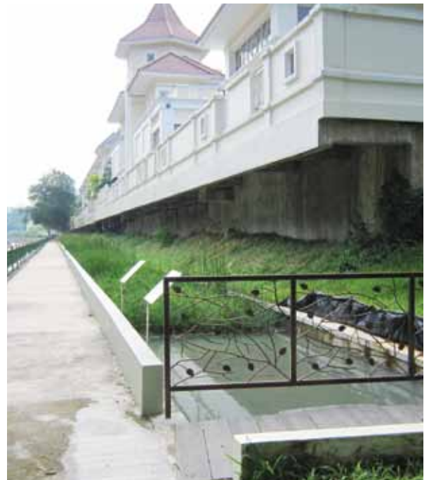
Fig. 4.33 Sedimentation forebay at Grove Drive
