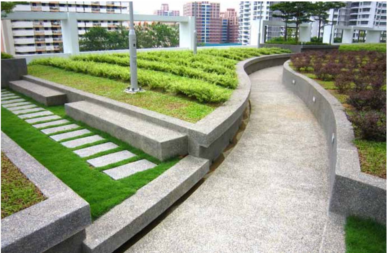
Fig. 10.13.1 Intensive green roof.
