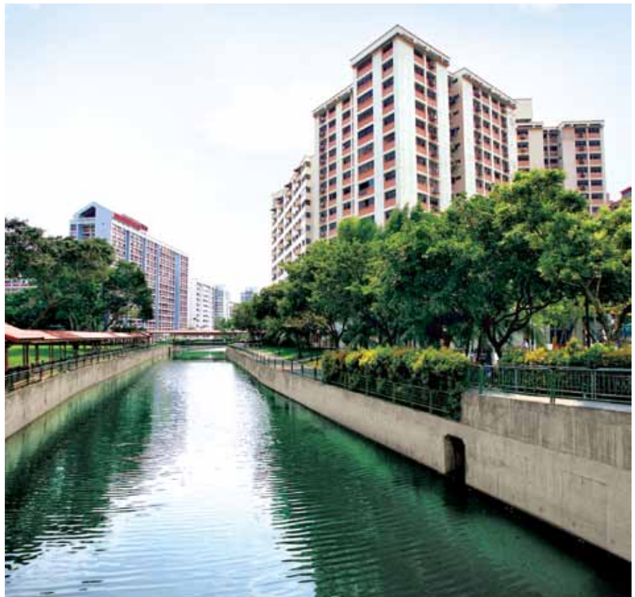
Fig. 2.1 Typical outlet drain (lined with concrete), an example of traditional stormwater management element.
