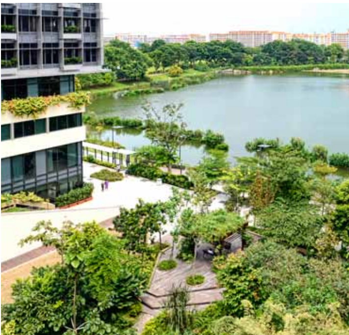
Fig. 4.32 Sedimentation basin at Yishun Pond is an aesthetic water feature next to Khoo Teck Puat hospital.
