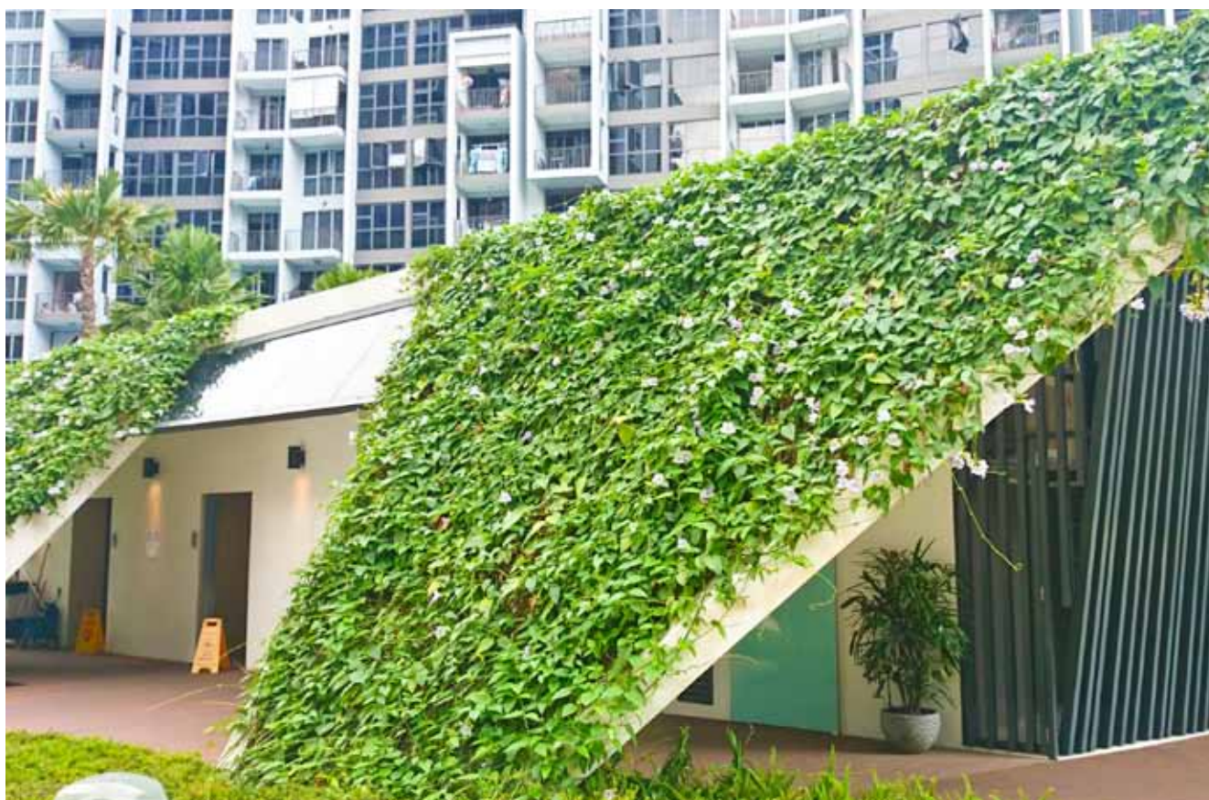
Fig. 10.7.3 Green roof at Club House.
