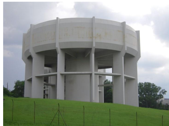
Fig 1b - Elevated tank
