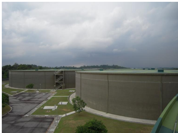
Fig 1a - Elevated tank
