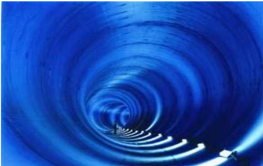
Tunnel Section of DTSS Phase 1
