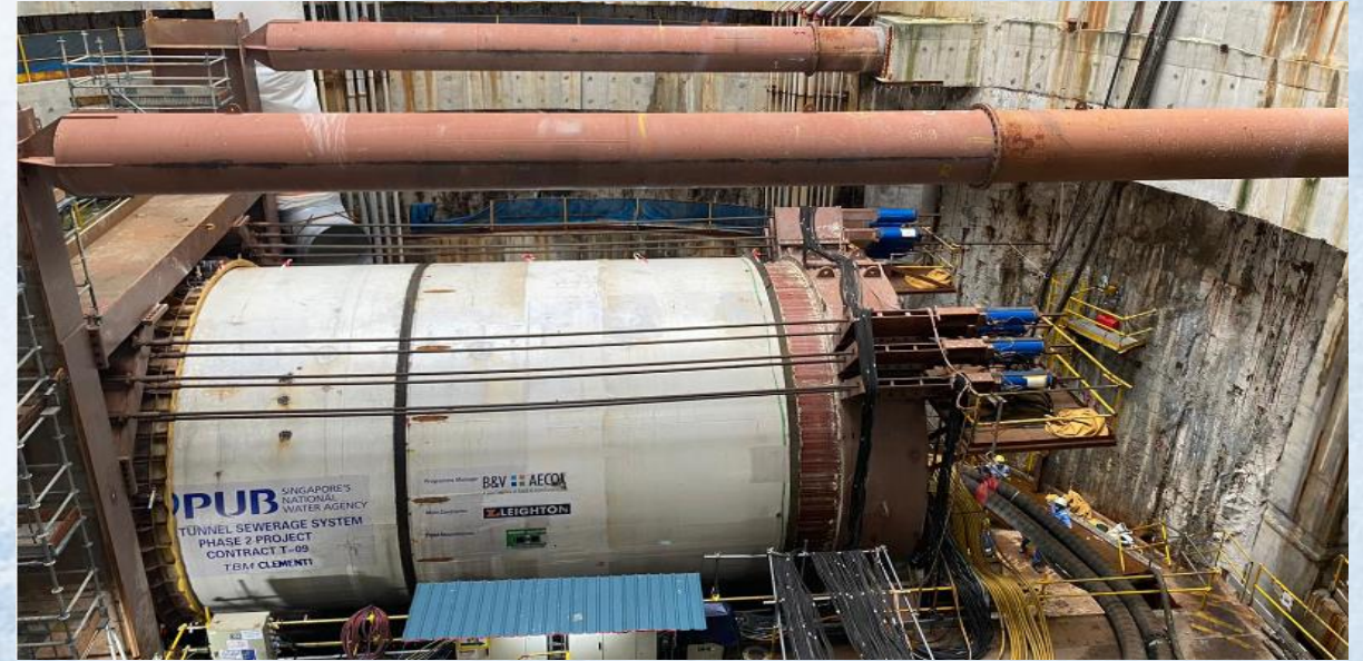
TBM Clementi in the starting position prior to the flying launch
