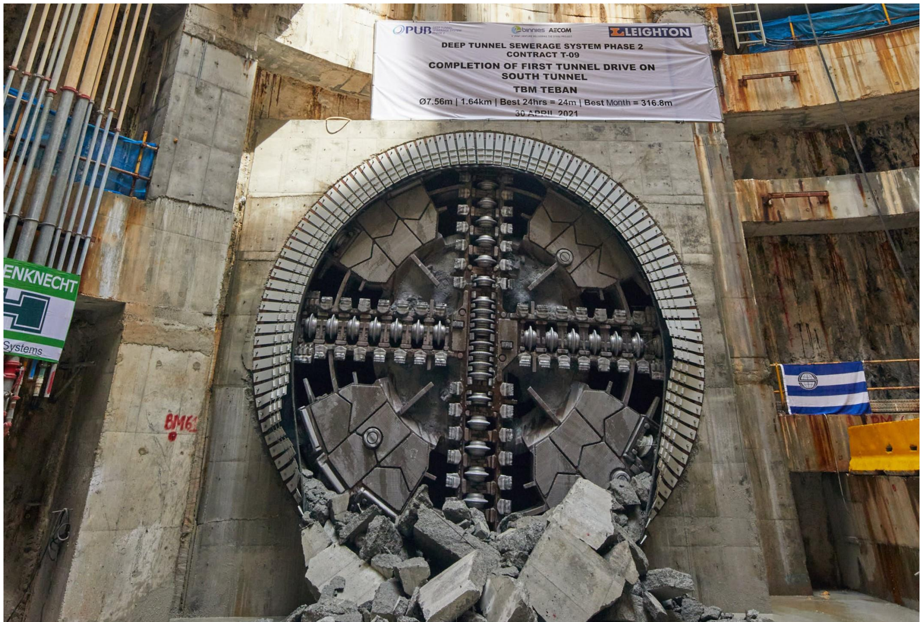
PHOTO: TBM TEBAN BREAKTHROUGH AT SHAFT N3 (INTERNATIONAL BUSINESS PARK)
