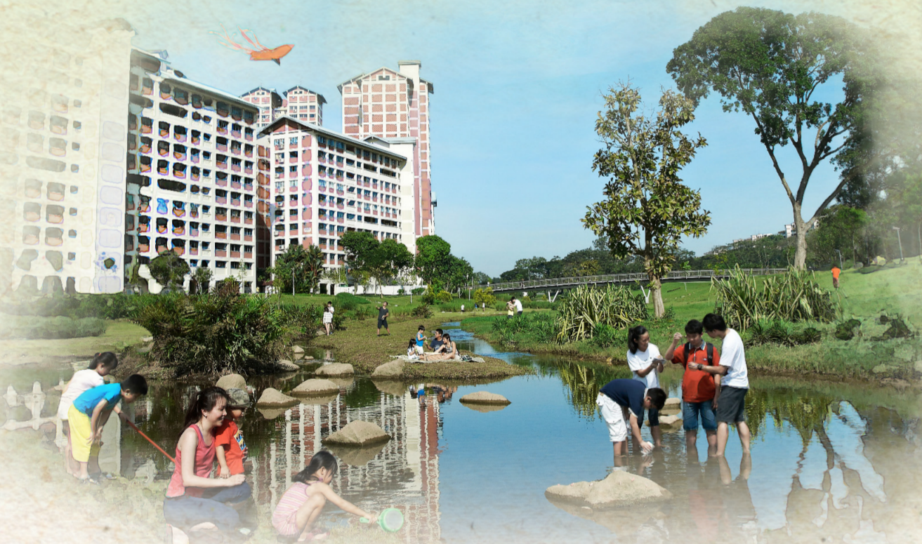
Transformation of a 2.7 kilometre-long concretised canal into a 3 kilometre-long naturalised river with bio-engineered river edges using a variety of plants and bedding materials. The naturalised river meanders through the park so park users can get closer to the water
