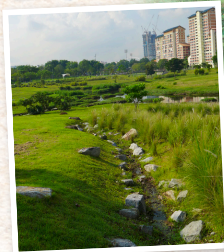
Gravel swales as part of the natural drainage system around the park
