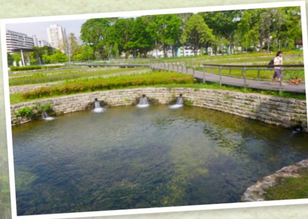
The Cleansing Biotope serves to treat water from the Kallang River and Landscape Pond. Clear, filtered water cascades from Cleansing Biotope into the Landscape Pond. This treated water is also channeled to the Water Playground after further UV treatment.
