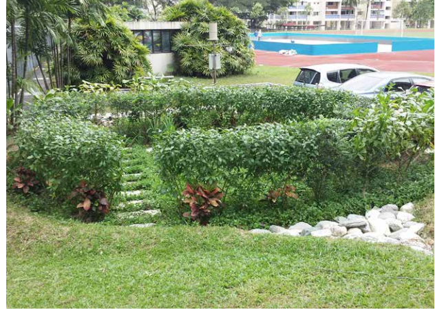
Fig. 2: Full-scale demonstration of a rain garden to improve runoff water quality
