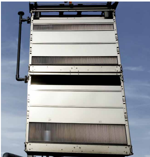
Fig. 1: A unit of the ceramic membrane used in the Upflow Anaerobic Sludge Blanket — Ceramic Membrane Bioreactor (UASB-CMBR) plant
