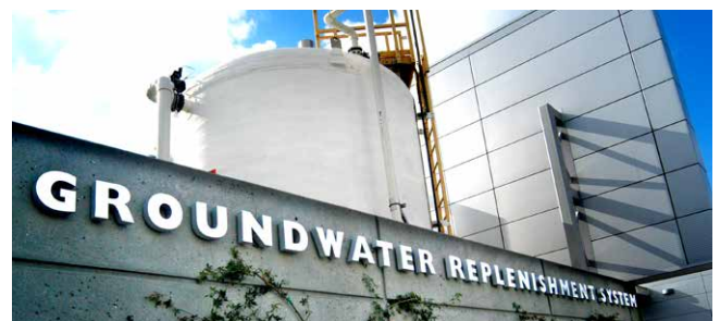
Fig. 2: Orange County's Groundwater Replenishment System Facility
