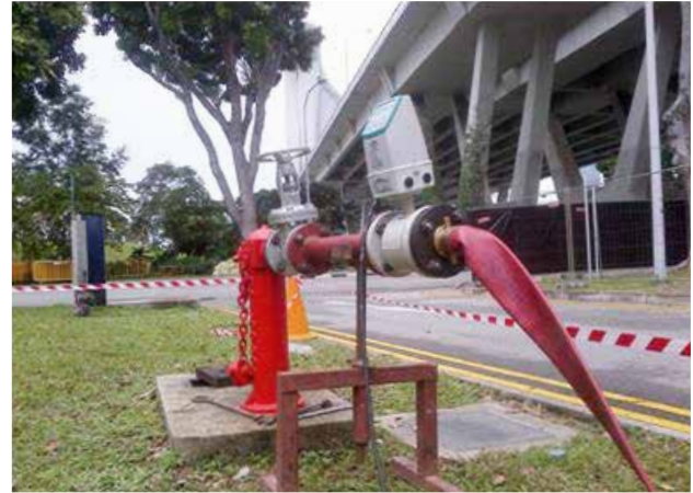
Fig. 2: Discharge set-up at a fire hydrant for simulating area leakage
