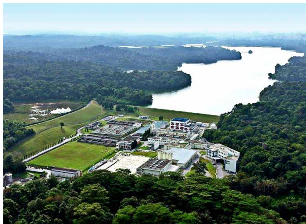
Fig. 2: Aerial view of Chestnut Avenue Waterworks, where the pilot trial of the P&T-GCMS system was conducted
