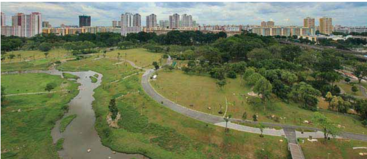
Figure 1.8 Acting both as a pathway and source solution along Kallang River, Bishan-Ang Mo Kio Park is an integrated multi-functional space that provides active recreational spaces for park users during dry conditions, but morphs into a floodplain during rain events, providing additional drainage capacity for the waterway.
