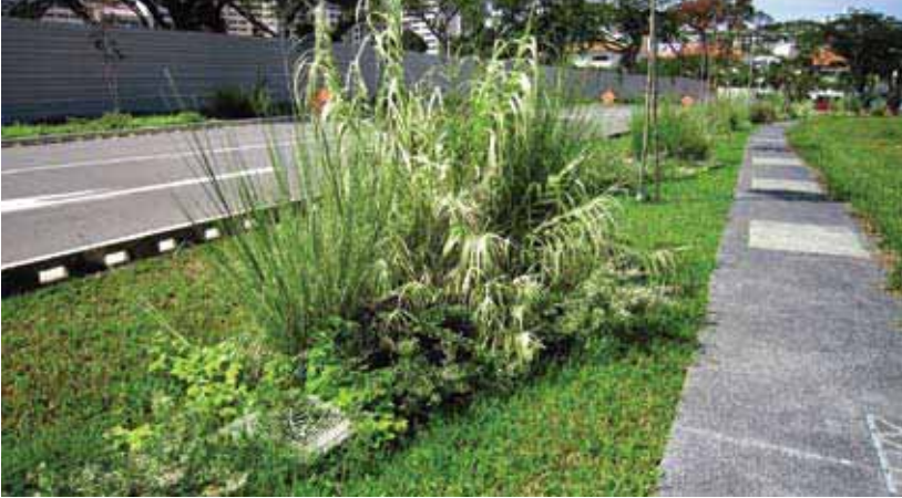
Figure 3.17 Bioretention swales along Margaret Drive.
