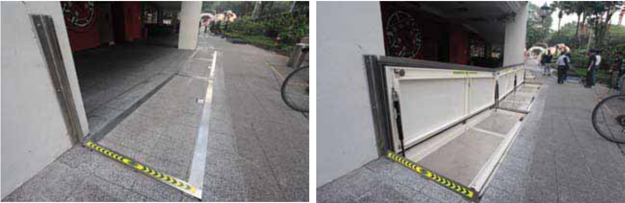
Figure 6.2.2 Flip-up barrier at the front of Tanglin Mall, in closed (left) and open (right) positions. This barrier was chosen to achieve seamless connectivity for pedestrians crossing the junction of Tanglin and Grange Road to Tanglin Mall.
