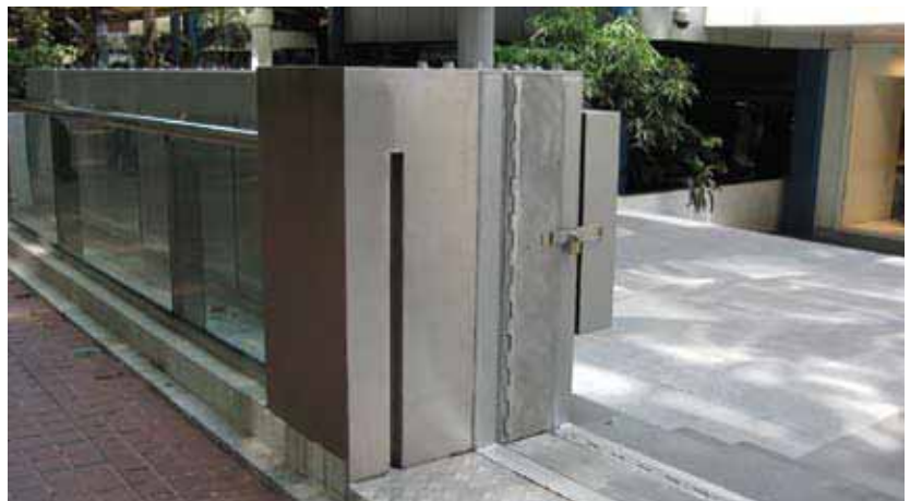
Figure 4.15 Sliding mechanical flood barrier system.
