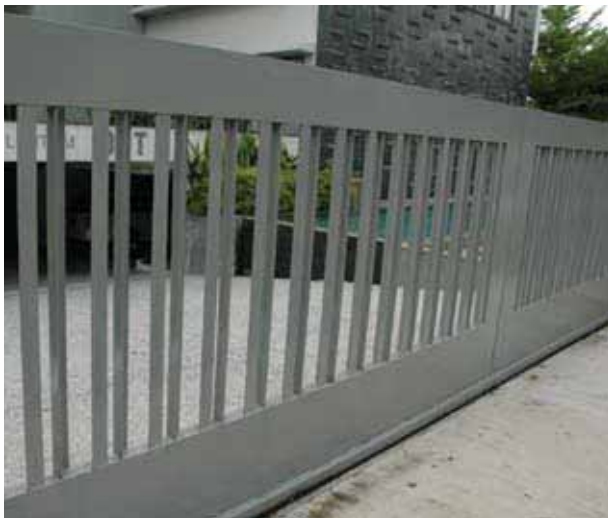
Figure 4.16 The entrance gate of this development leading directly to the basement car park was designed with a solid bottom section, with openings (for aesthetics) starting at the level above the required minimum crest level. A cross-section schematic of the gate is shown on the right.
