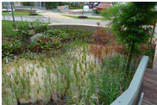
Figure 5.4 A low seat wall, together with clear signage, can be used to limit access into the bioretention feature.
