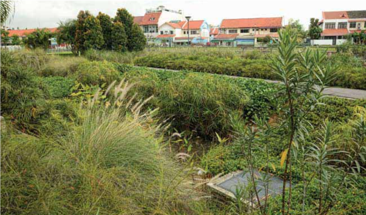
Figure 3.14 A bioretention basin at Balam Estate with an overflow pit.
