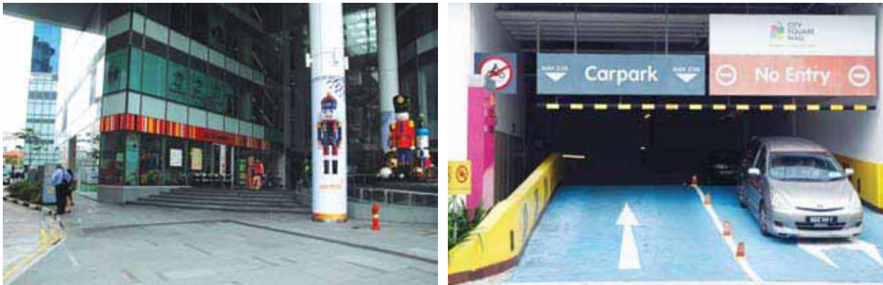
Figure 4.1 Minimum platform levels for developments and crest levels for entrances to basements are some examples of structural receptor solutions.
