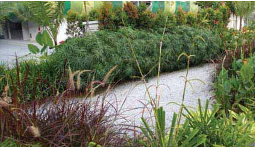
Figure 3.18 Example of a gravel trench serving as a conveyance channel for stormwater runoff.
