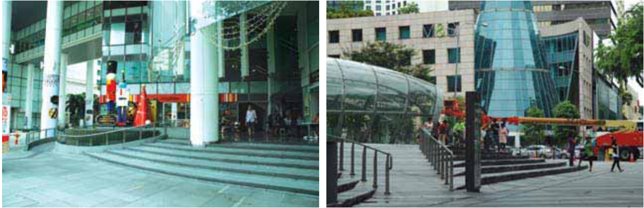
Figure 4.3 Steps and ramps are some of options to achieve the minimum platform levels for developments with entrances to underground facilities.
