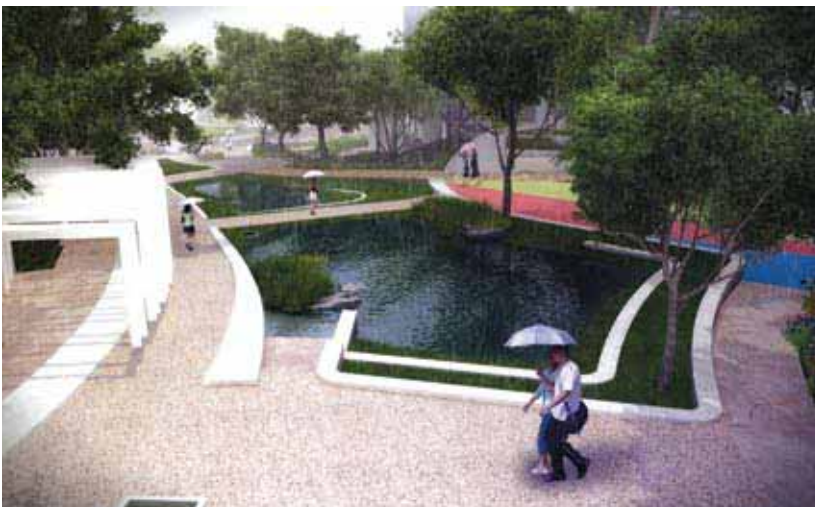
Figure 6.1.5 Bioretention basin serving as a multi-purpose lawn during dry weather. During a rain event, it acts as a temporary detention feature for stormwater runoff.
