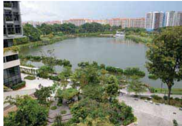
Figure 3.6 Yishun Pond, a stormwater retention pond adjoining Khoo Teck Puat Hospital.
