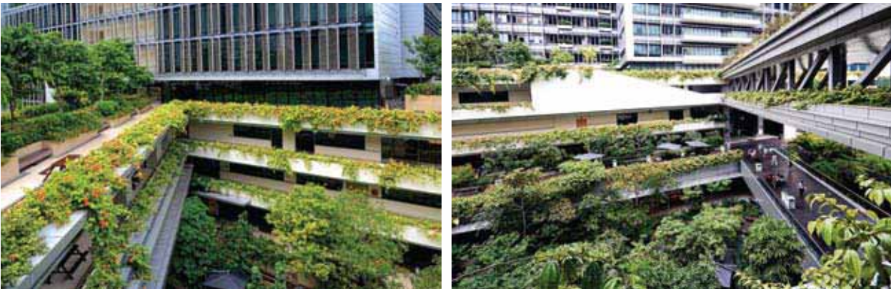
Figure 3.10 Planter boxes on the sides of the building and along pedestrian bridges at Khoo Teck Puat Hospital.
