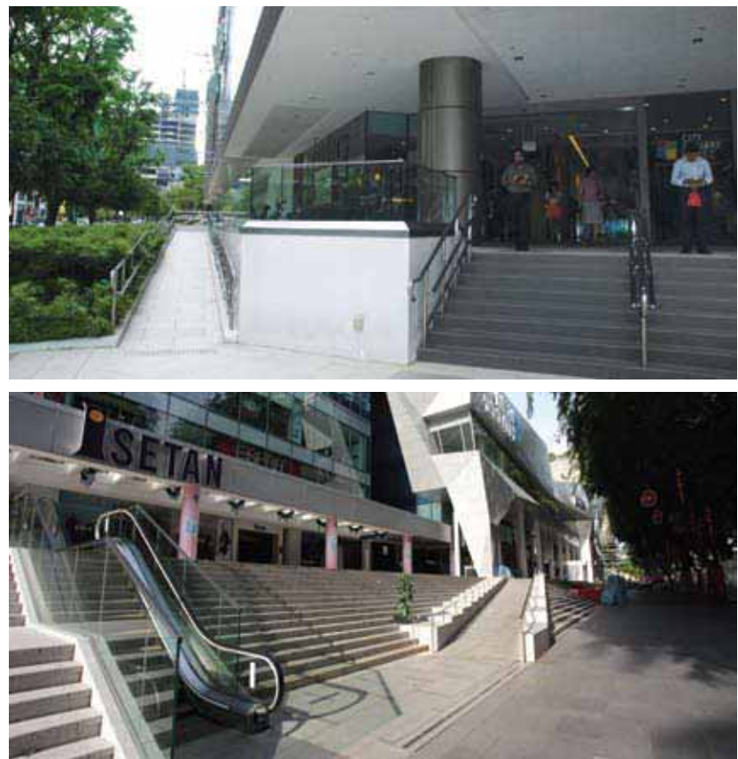
Figure 4.10 Two examples of staircases and ramps used to bridge the level differences between ground levels and the development’s platform level.
