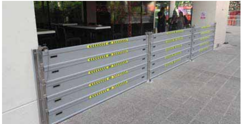
Figure 4.13 Manually installed slot-in barrier system.
