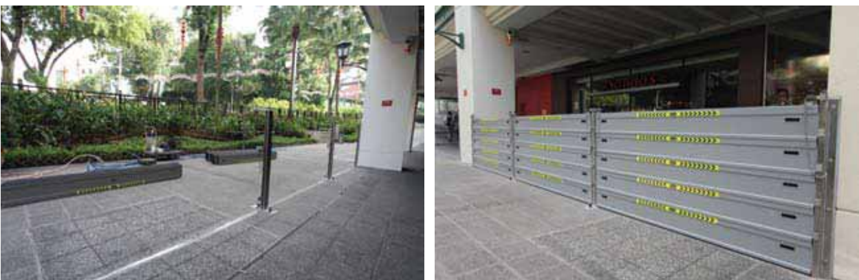
Figure 6.2.4 A multi-slot barrier at the front of Tanglin Mall before (left) and after (right) installation. These barriers have to be installed manually.
