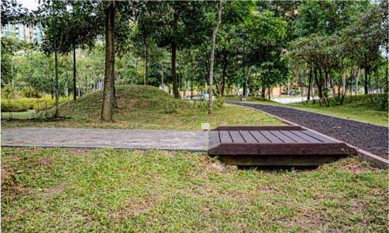
Figure 5.1 A crossing installed across a grass conveyance swale ensures a smooth transition between the two walkways, and also protects the soil beneath from being compacted by pedestrians, which would otherwise reduce the infiltration capacity of the swale.
