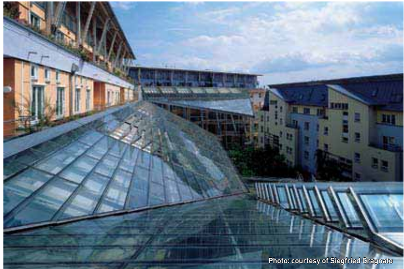
Figure 6.4.2 Rainwater from the entire roof area (approximately 4000 m 2 ) is collected and channelled into the cistern. Approximately 70% of the cistern serves as stormwater detention storage, 17% of the storage is used for emergency purposes (fire-fighting), and 13% is used to circulate rainwater throughout the building as “natural air-conditioning”.
