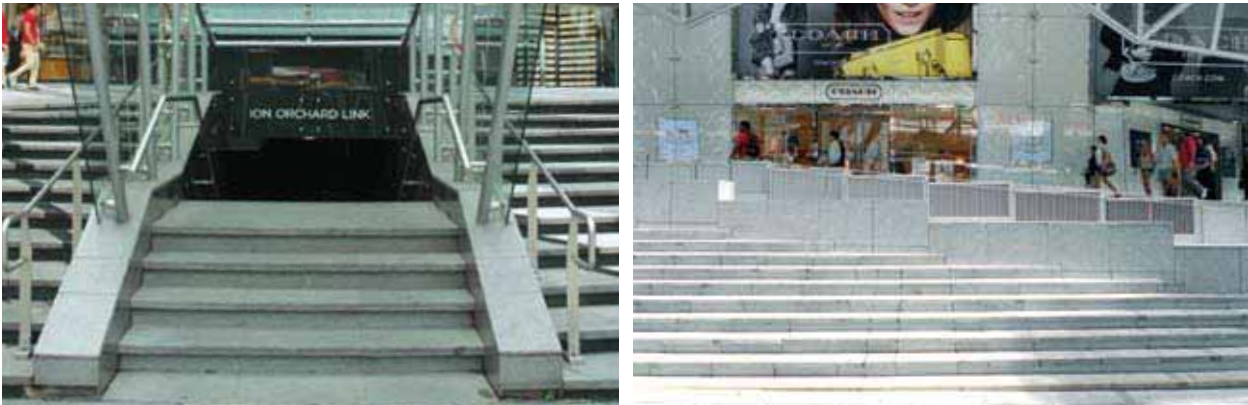
Figure 4.4 Additional crest protection levels are required for developments with underground linkages to MRT stations (e.g. Ion Orchard Link) and for all openings to basement facilities, including ventilation ducts (e.g. Wisma Atria)
