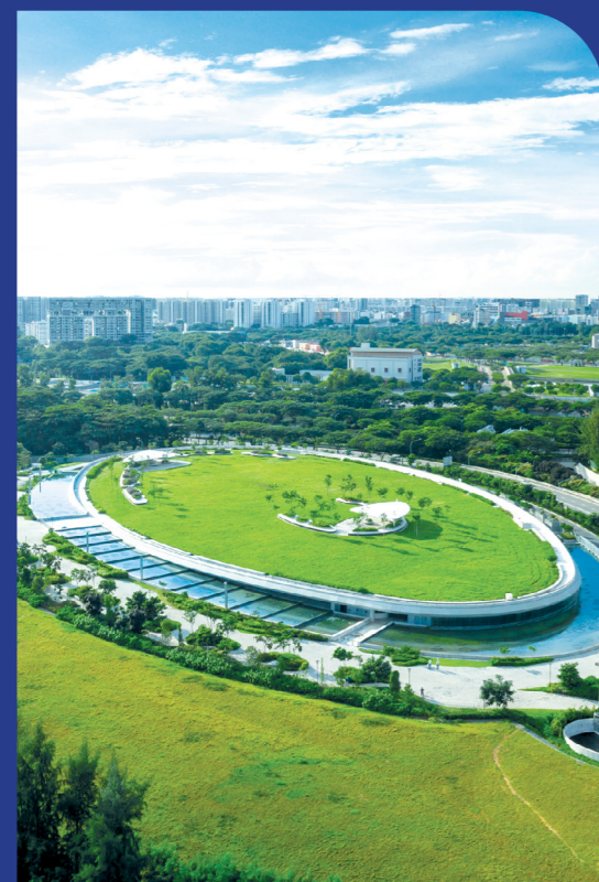
Aerial view of Keppel Marina East Desalination Plant. (Photo credit: Keppel)
