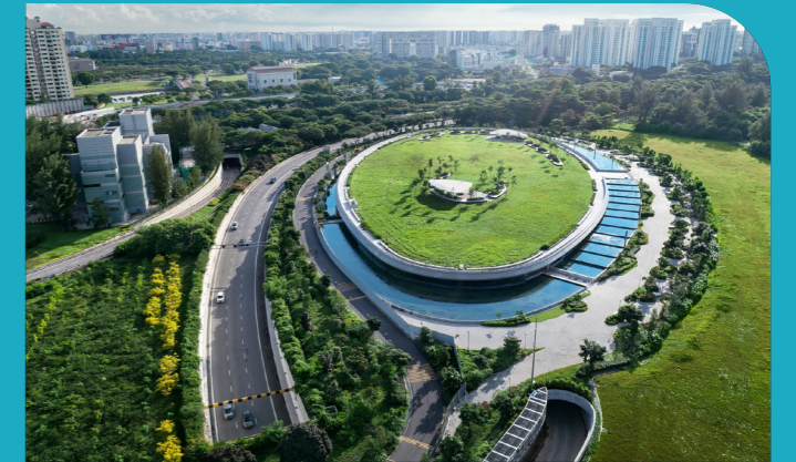
Aerial view of Keppel Marina East Desalination Plant. (Photo credit: Keppel)
