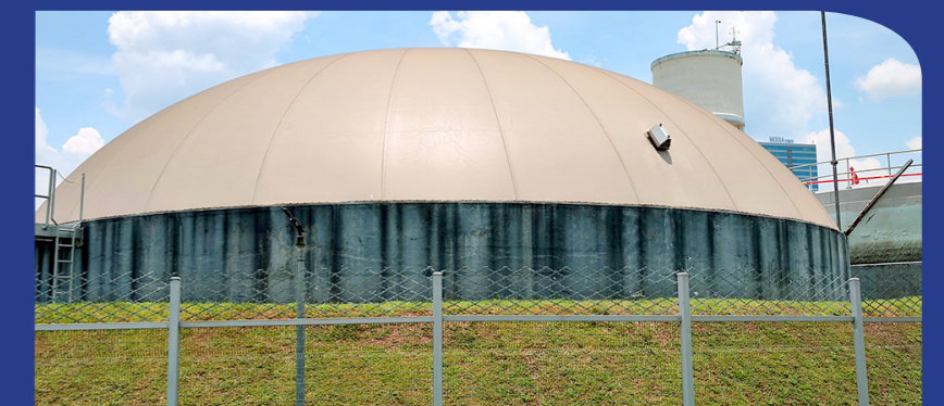
Biogas holder at Ulu Pandan Water Reclamation Plant.
