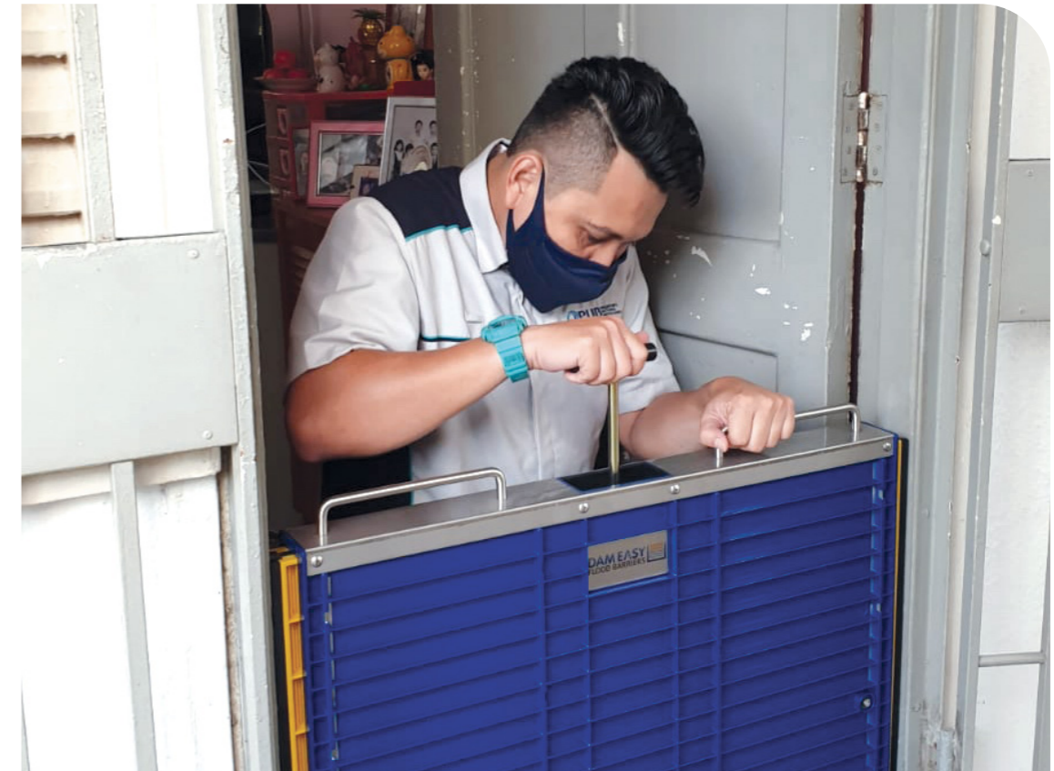
A PUB officer helping a resident to install a flood barrier.
