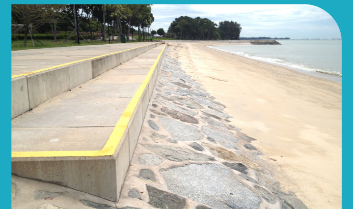
Composite stepped revetment, as seen along East Coast Park.
