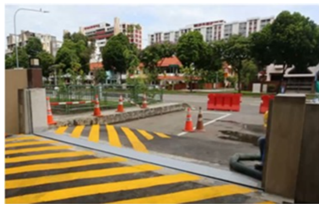
Before Activation: Automated Flood Barrier (AFB) at Fortune Park
