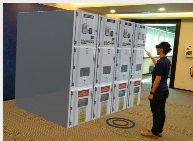
Training how to operate & maintain equipment through Mixed Reality technology
