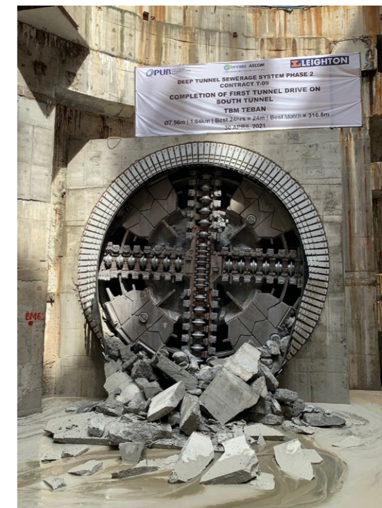
Tunnel Boring Machine Teban Breakthrough in South Tunnel
