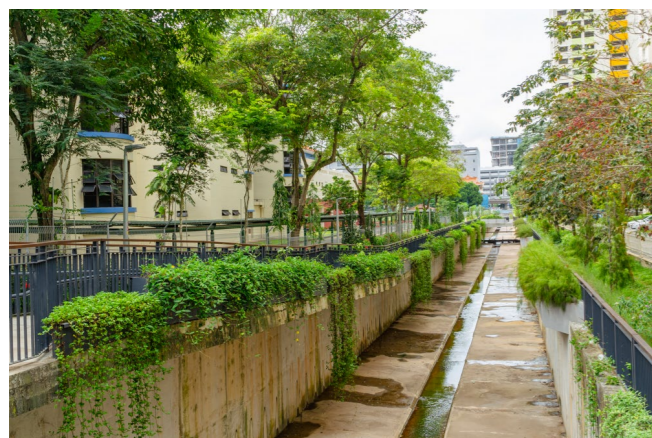
Completed Alexandra Canal subsidiary drainage work
