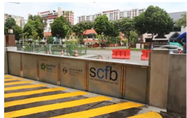
Fully Activated: Automatic Flood Barrier (AFB) at Fortune Park
