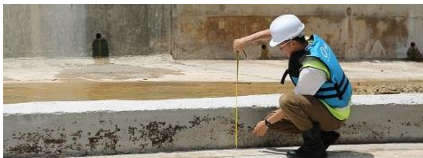
PUB engineer Jeremy Tan checks works at a construction site to ensure that
