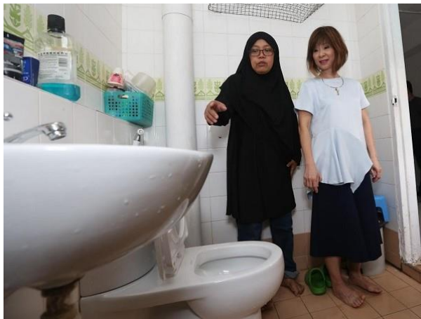
Above: SMS Dr Amy Khor sharing the benefits of a water efficient water closet with a resident.
