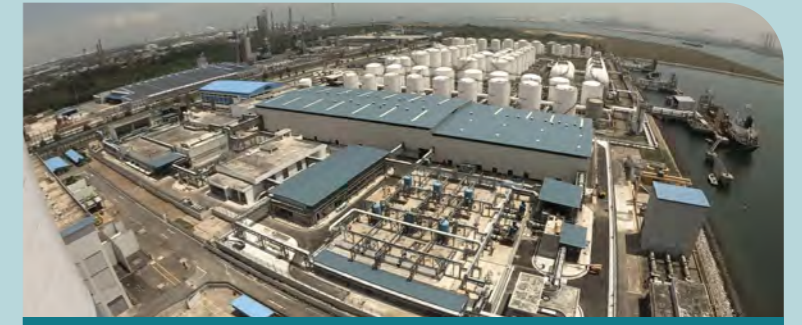
An aerial view of the Jurong Island Desalination Plant. (Photo: PUB)
