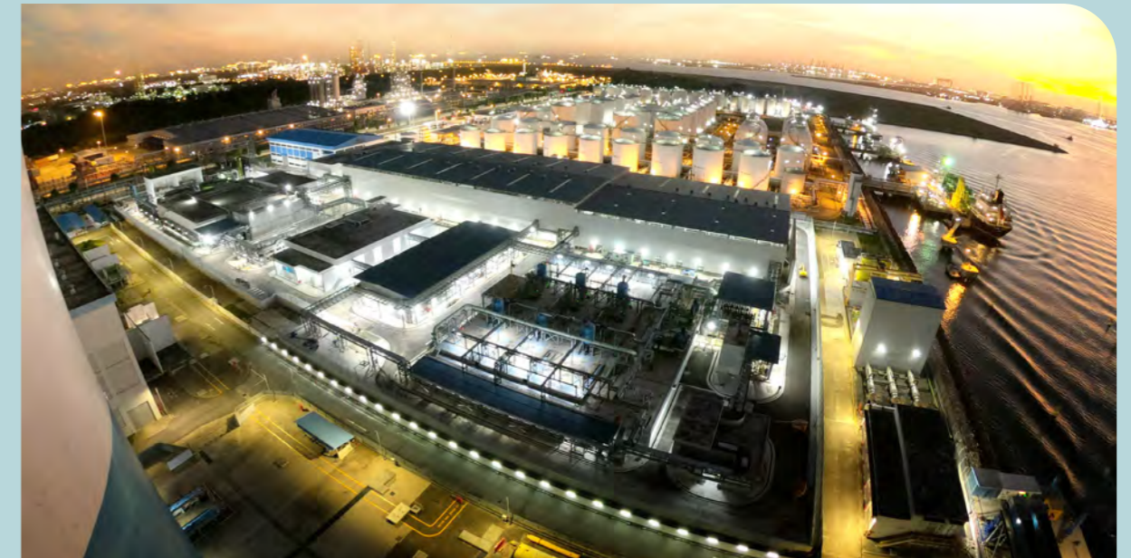
An aerial view of the Jurong Island Desalination Plant. (Photo: PUB)
