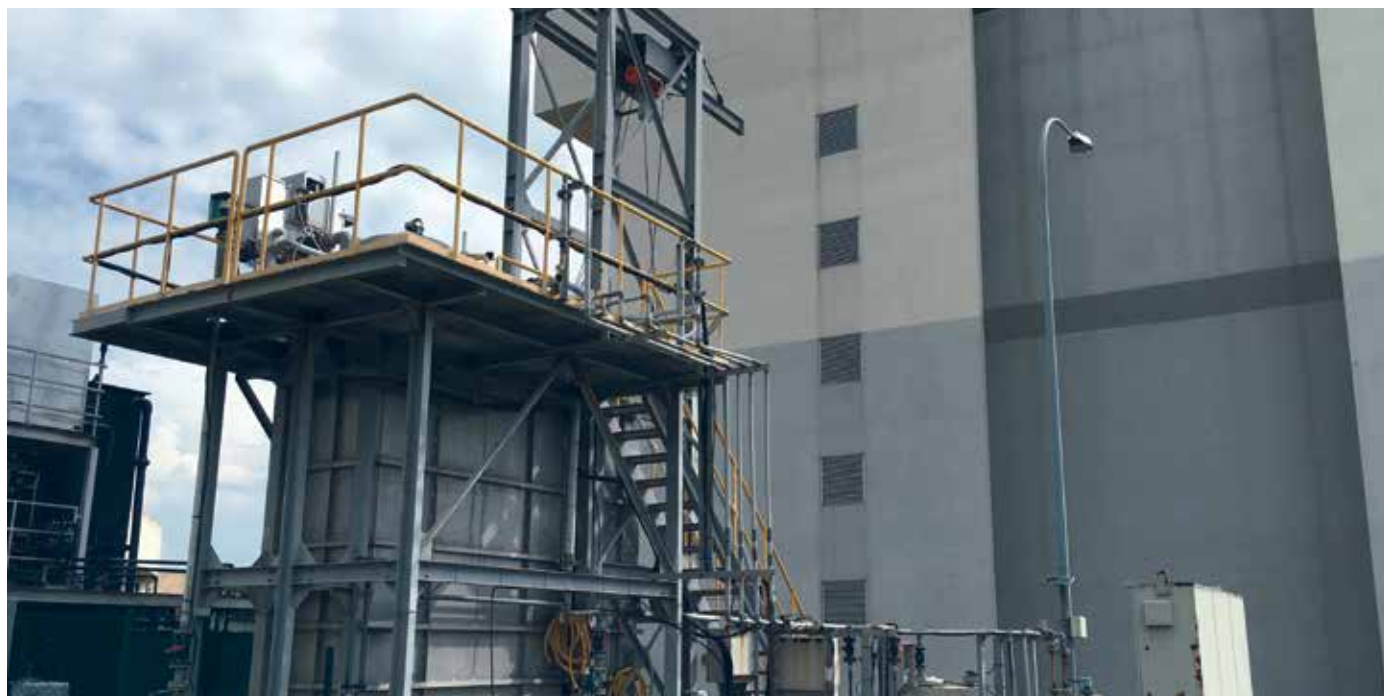
Fig. 1: A pilot-scale MBR system being evaluated in the study
