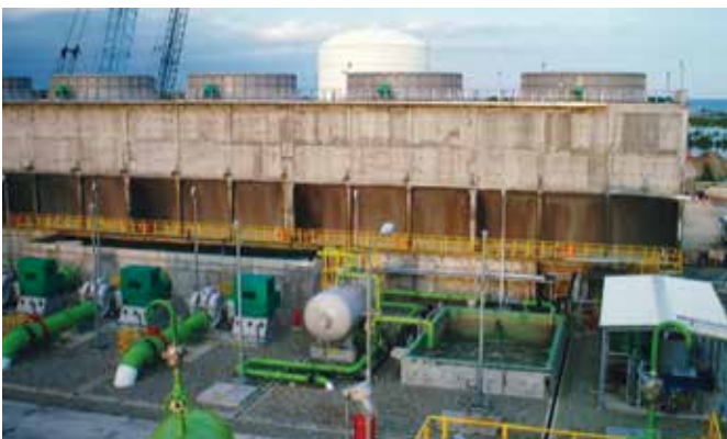
Fig. 1: MHI-AP's seawater cooling tower system, currently in operation in Indonesia
