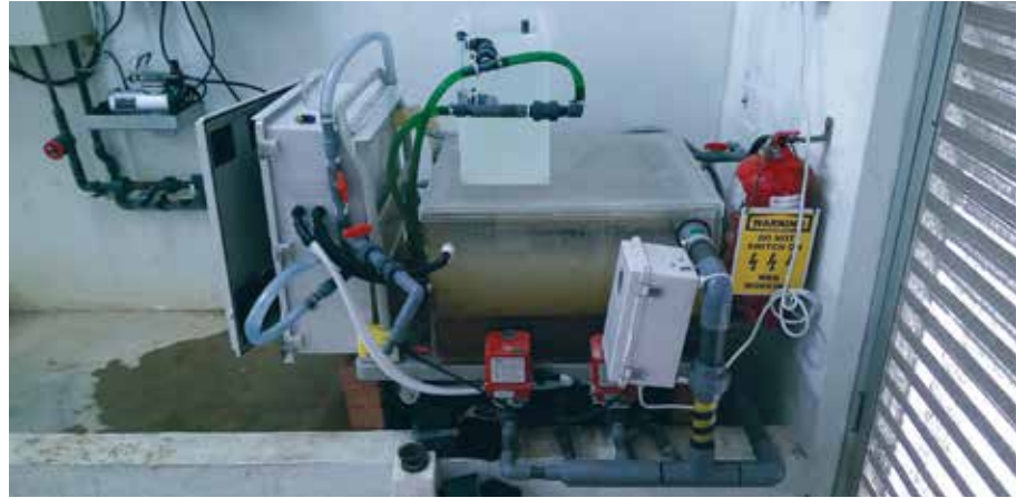
Fig. 2: Pre-filtration module of FAMS Gen2 with backwash mechanism for test-bedding at JRWW
