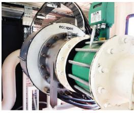
FIG. 2: Algae control unit (ACU) installed along the pipeline
