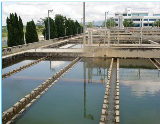
Fig. 1: A section of the Johor River Waterworks
