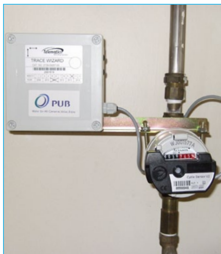
Fig. 1: An automated water meter that monitors residential water use in Singapore
