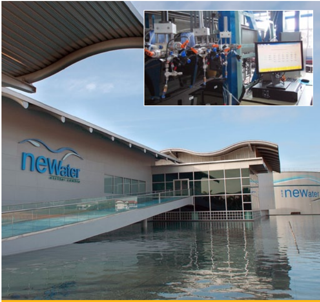
Bedok NEWater Factory houses a number of projects related to Membrane Technology, such as the Membrane integrity sensors
