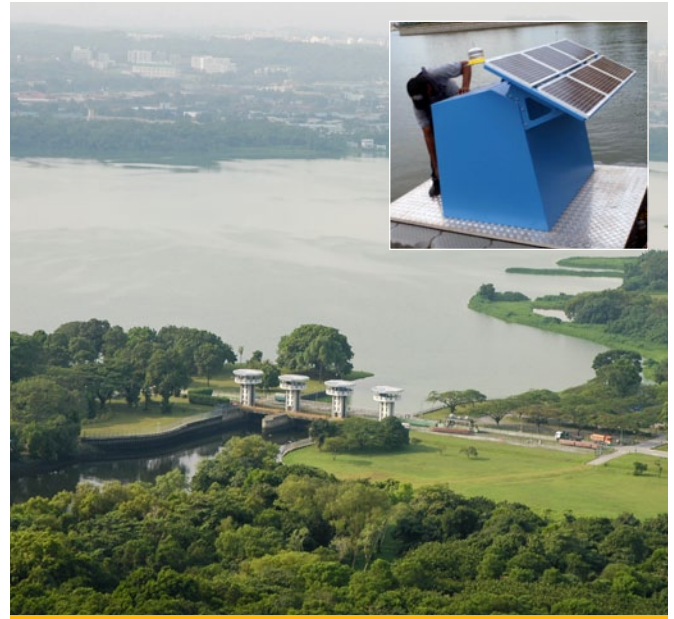
Real-time water quality monitoring and modelling are conducted at Kranji reservoir
