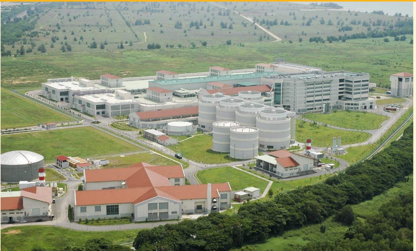
PUB's Water Reclamation Plants, such as Ulu Pandan WRP (top) and Changi WRP (bottom), offer test-bedding sites for used water treatment projects
