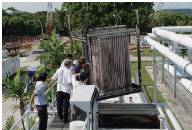
Fig. 2: PUB personnel inspect an MBR cassette at one of the Bedok pilot plants
