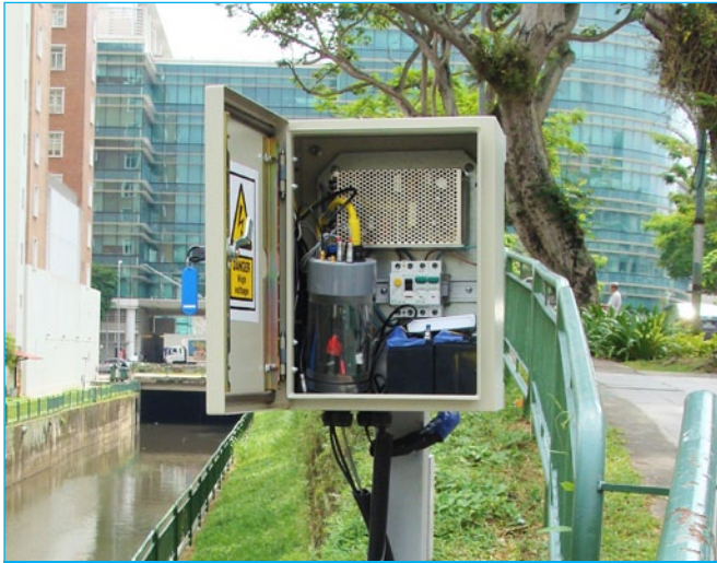
Fig. 1: Singapore's central business district is now home to a network of wireless sensors that continually monitor the water distribution system
