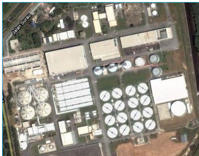
Fig. 2: Overview of the Kranji Water Reclamation Plant
