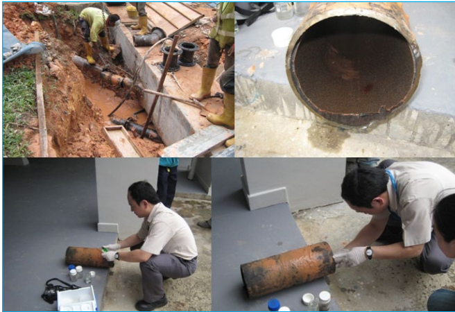
Fig. 1: Researchers collecting samples from a pipeline at Yishun in Singapore
