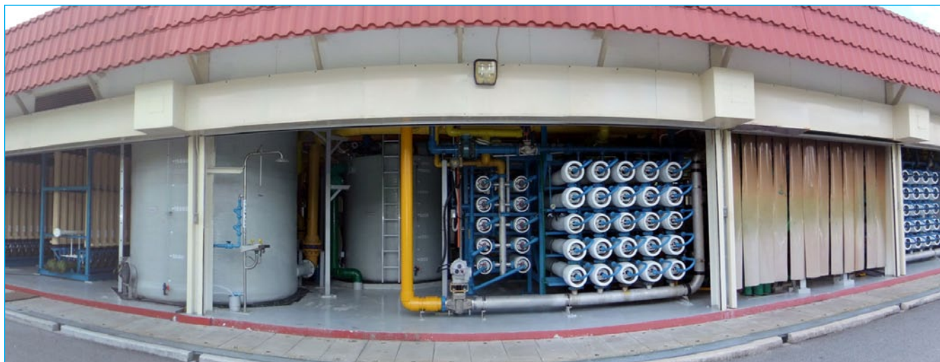
Fig. 1: The variable salinity process enables treatment of both brackish and seawater at the same facility, allowing the catchment area to increase to more than 90% of Singapore's land area.
