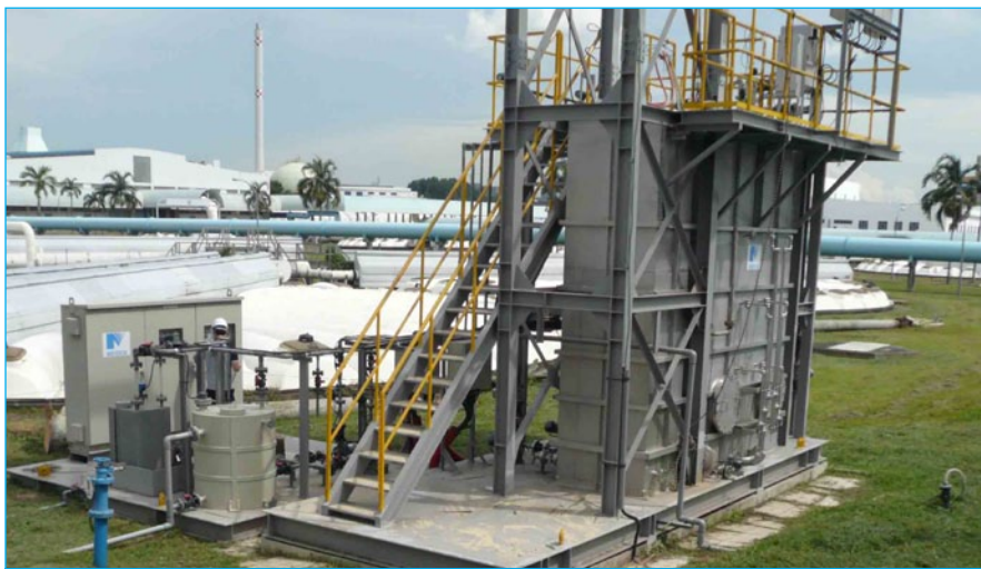
Fig. 2: The ceramic MBR pilot plant
