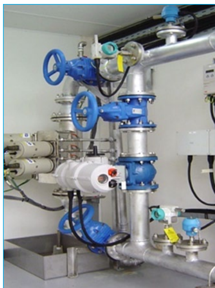
Fig. 1: The ultrasonic reactor for breaking down sludge prior to microbial processing
