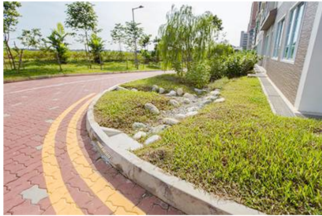
Figure 5.12 Energy Dissipator at swale inlet
