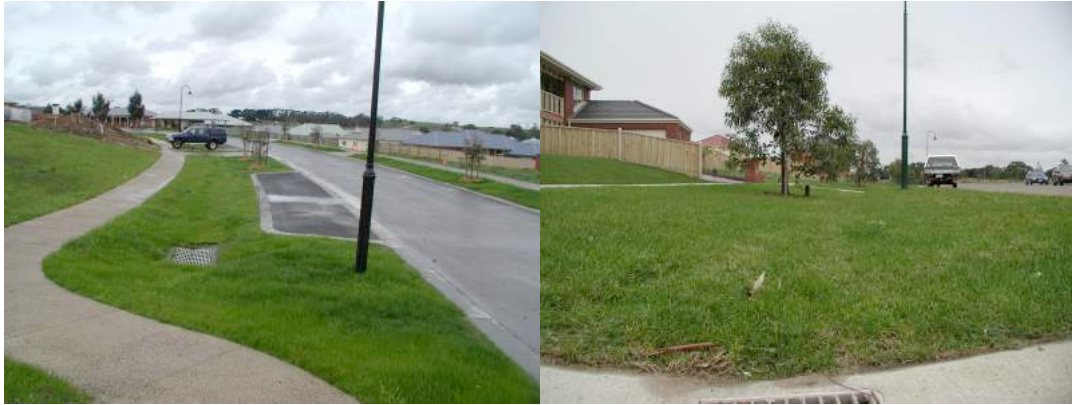
Figure 5.15 Similar buffer swale system for conveying runoff
