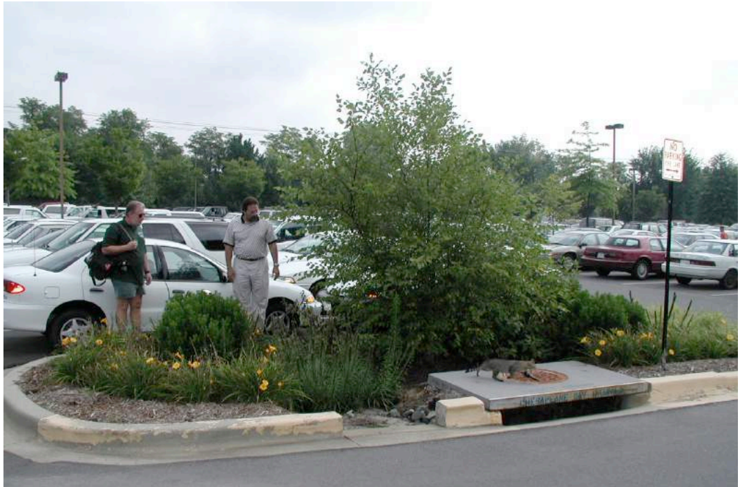
Figure 7.13 A conventional side entry pit for overflow from Bioretention Pod. Once inundated to street level, stormwater will no longer enter the bioretention raingarden but will instead be conveyed to the adjoining side entry pit.
