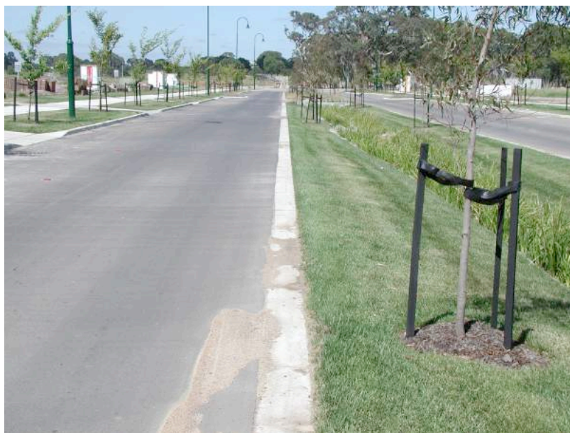
Figure 6.10 Flush Kerb without Setdown, showing Sediment Accumulation on Road
