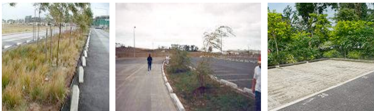
Figure 6.9 Kerb Arrangements with Breaks to Distribute Inflows on to Bioretention Swales and Prevent Vehicle Access
