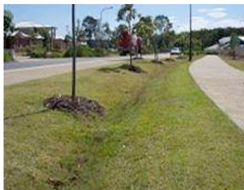
Figure 5.4 Swale incorporated into road reserve
