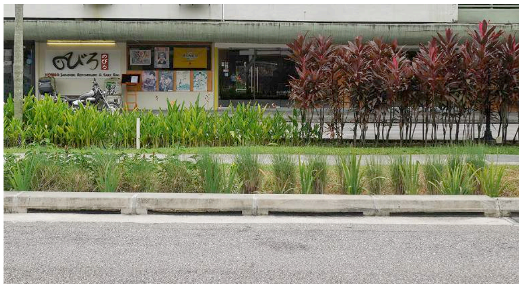
Figure 7.15 Example of a bioretention system in a street (Faber Hill Estate)
