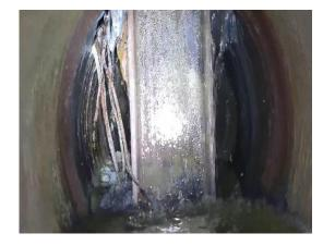
Pile punctured a sewer pipe causing sewer to surcharge. This work was carried out near the sewer pipe without approval from PUB.
