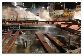
Necessary support structures not installed for the water pipe, as stipulated in the procedures for carrying out excavation work. This resulted in the water pipe being dislodged at its joint.
