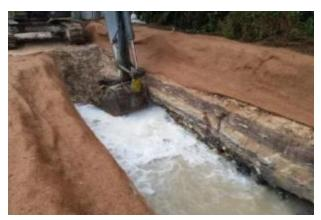
Tip of the excavator bucket punctured a water pipe at the construction site. This work was carried out within the vicinity of water pipe without approval from PUB.
