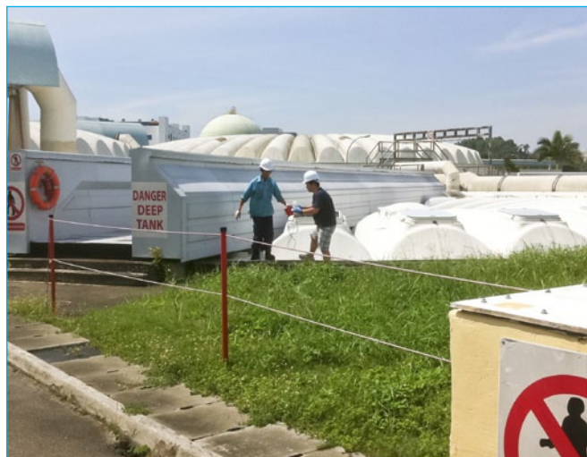
Fig. 2: Singapore's Ulu Pandan Water Reclamation Plant
