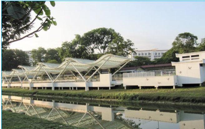
Fig. 1: The Aquatic Science Centre at Sungei Ulu Pandan, Singapore, is a state-of-the-art green building that facilitates research into, and promotes public awareness of, urban water management
